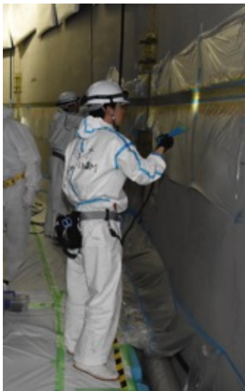
Seal whole welding lines
