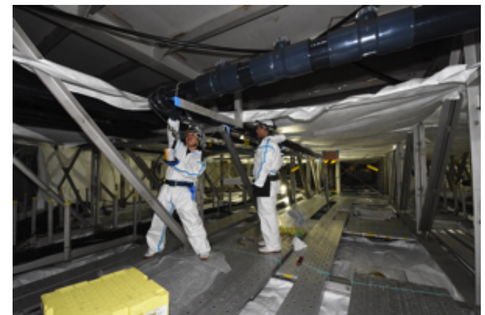
Install new water pipe
