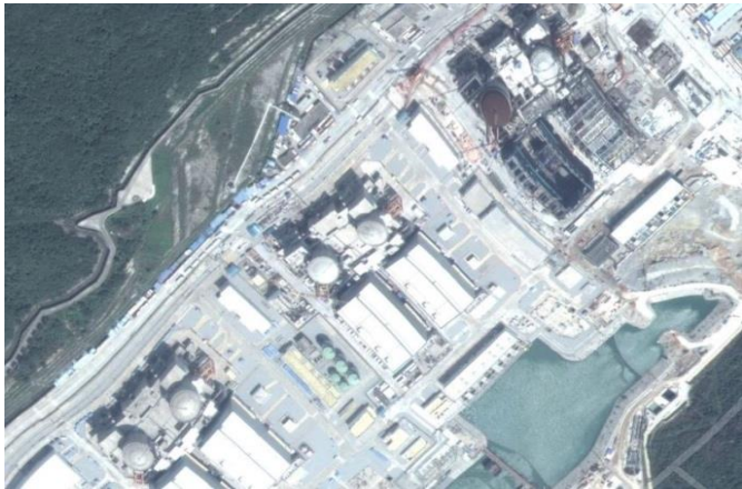
Yangjiang Power Plant
