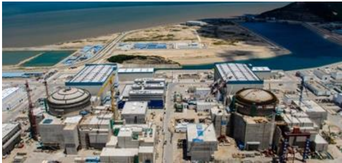
Taishan Power Plant
